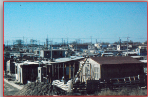
© Research Archives, 2014, In situ builders
