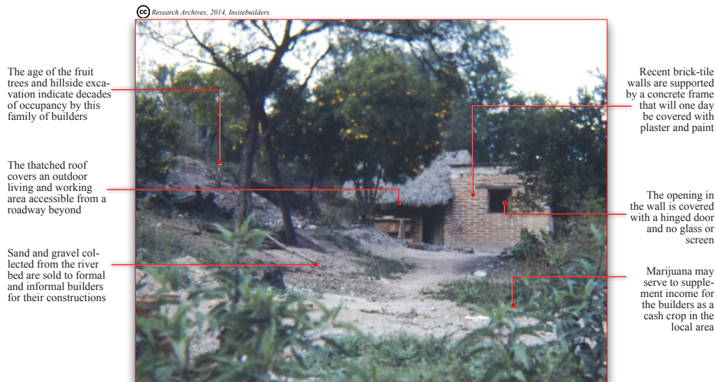
Beginning slowly, a homebuilt house evolves according to the well being of its builders and a fading threat of eviction. In time, ongoing improvements reinforce open and obvious possession and strengthen a claim as adverse landholders.
